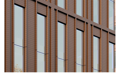
Facade Neighborhood Context
