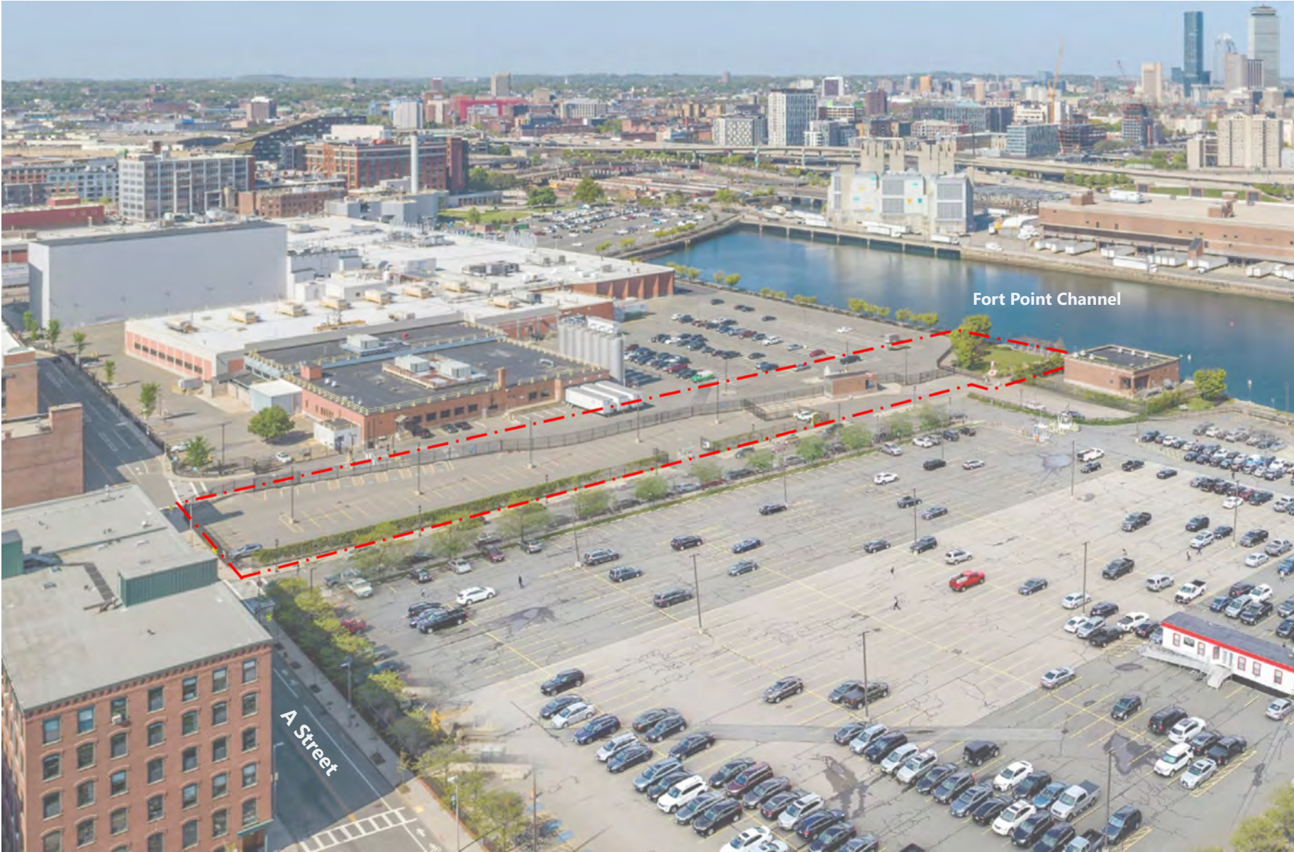
Figure 1.4 Aerial View - Existing Conditions
